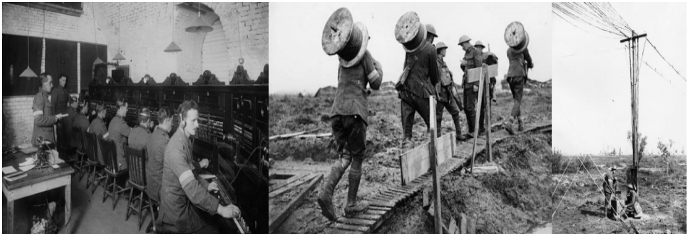
(left) telephone exchange operators. (centre) Line carried forward. (right) Air Line being erected
